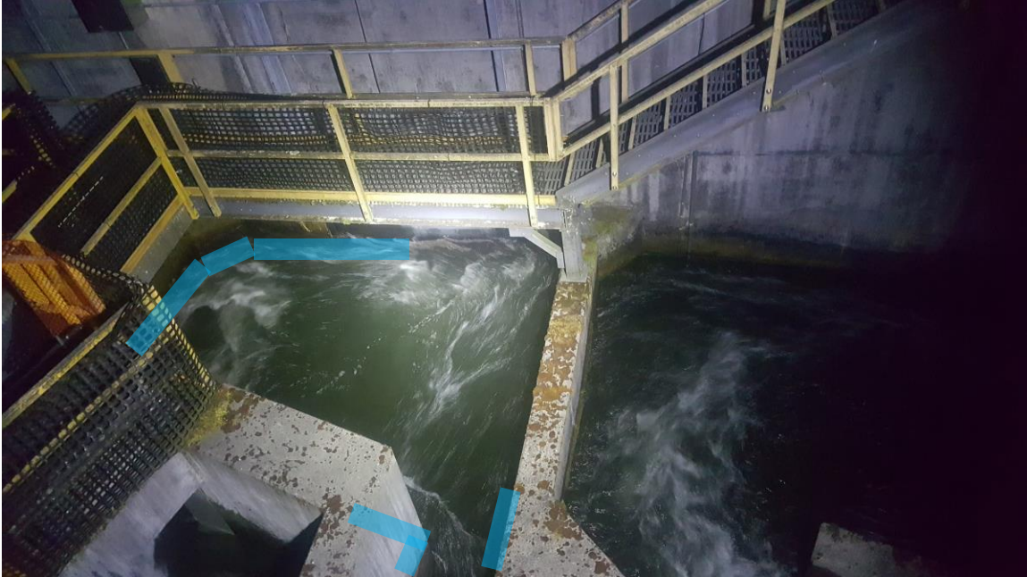
Figure 4. Photo of the serpentine weir fishway during night time tour on July 11, 2018. The blue lines represent areas where the placement of pucks is expected to help adult lamprey passage. Several lamprey can be seen attached to the wall near the water surface in the center of the picture in the high flow high turbidity section.
