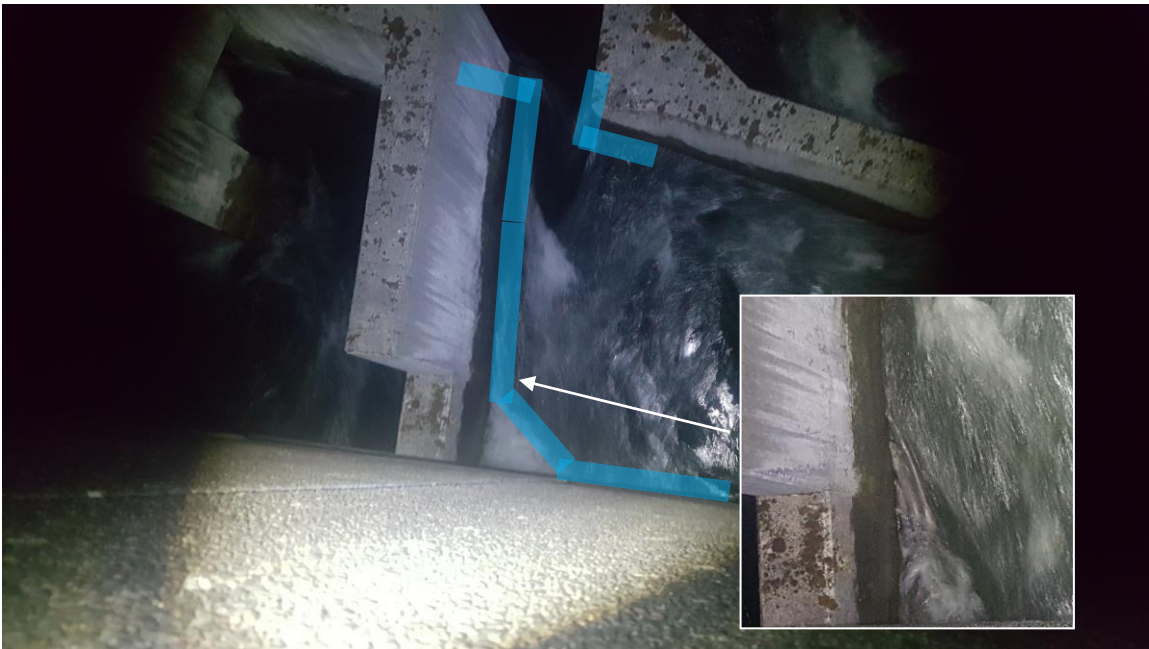
Figure 5. Photo of another section of the serpentine weir fishway during night time tour on July 11, 2018. The blue lines represent areas where the placement of pucks is expected to help adult lamprey passage. Several lamprey were observed attached to the wall as shown in the inserted photo.
